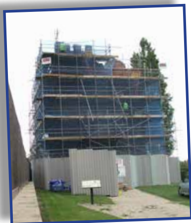
Repair work being carried out
