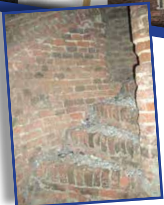
The staircase at Hussey Tower before the repair project
