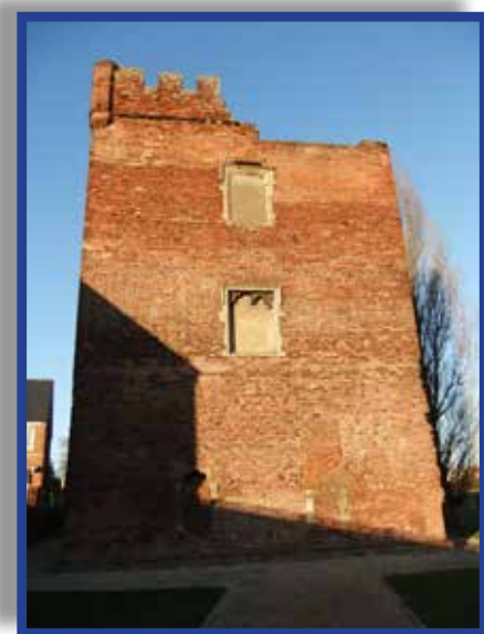
The finished repairs
